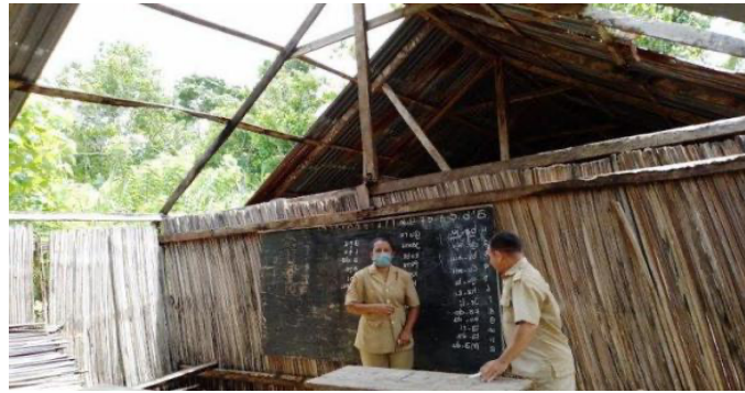
Emergency building of State Elementary School Nunka in Ponain Village, Amarasi Sub-district.
